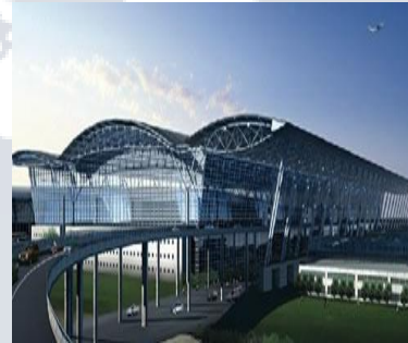
Pudong Int. Airport
